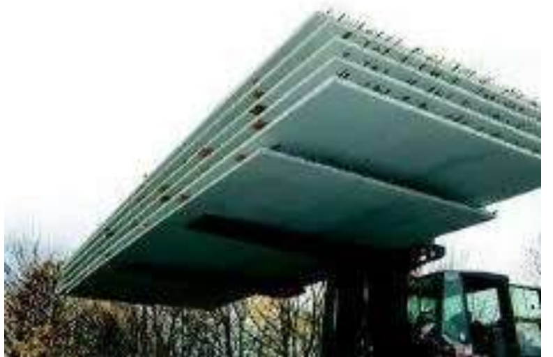
Transport der Filigree deiling transportation tot he storage area
