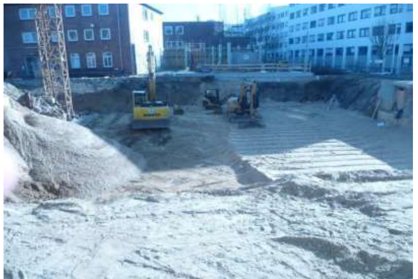
Construction works of building 25 from the perspective of building 26.
