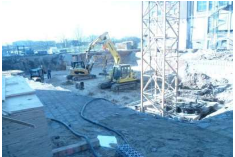
construction works of the new buildings 25
